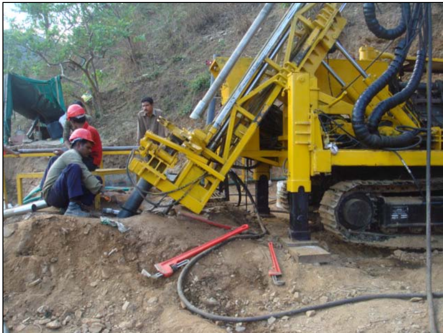
DDH-10AA018 setting collar pipe, May 8, 2010. Hole is inclined at -58^\circ .
